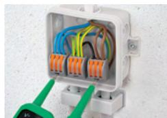
Testing via Profi-LED+ voltage tester (206-806).
